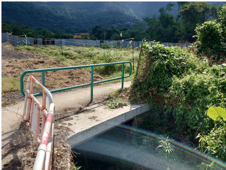
Plate 5. Covered portion of CH.B0.00 – CH.B149.77 on 22 November 2023.
