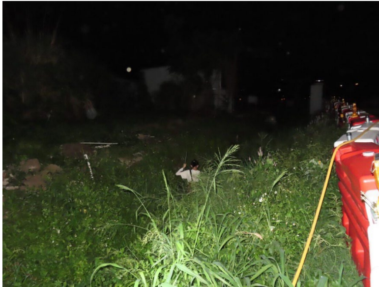
Plate 4. Site condition of CH.B0.00 – CH.B149.77 on 18 April 2024.
